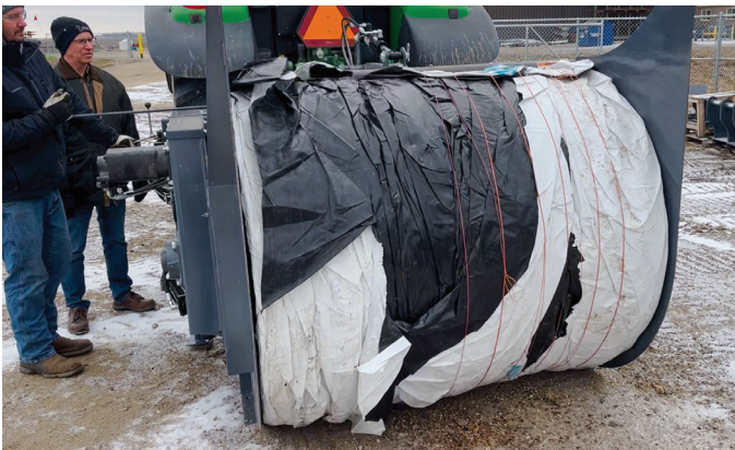
Turn for Tying & Discharge
